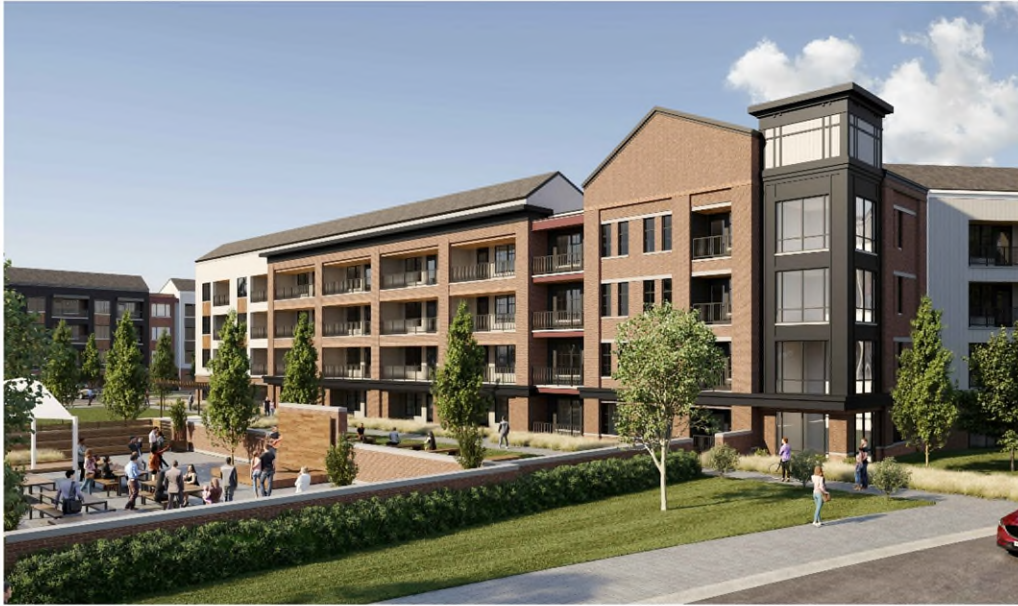
View of Building 2 Looking South-East from Kincaid Blvd
