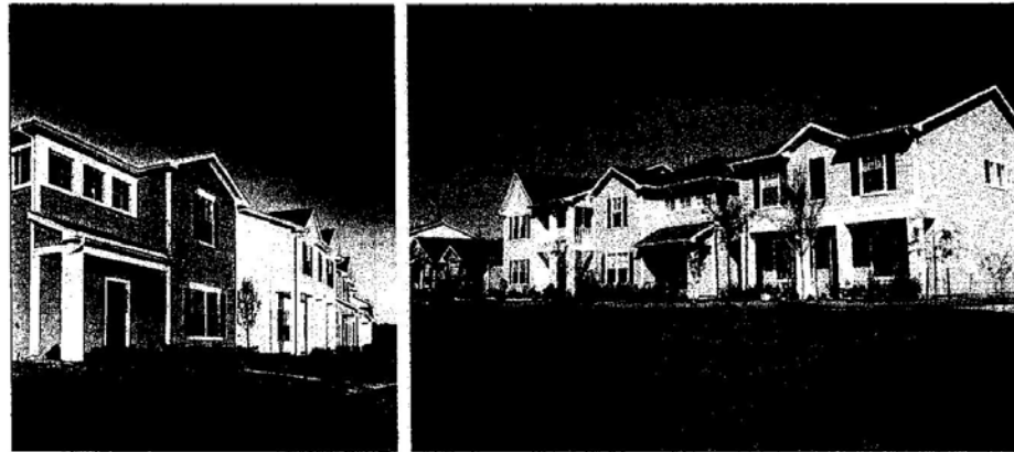
Photos: Parkside, Houston, Texas
