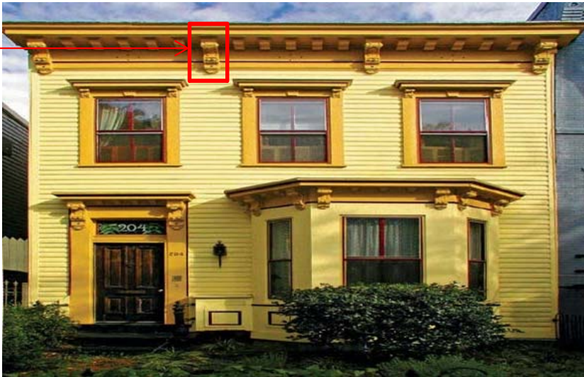
Decorative brackets at eaves/cornice
