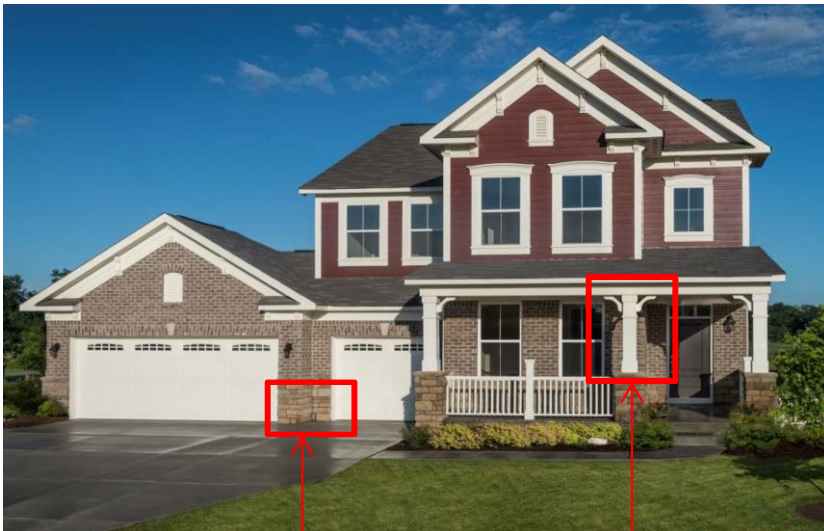
Masonry water table
