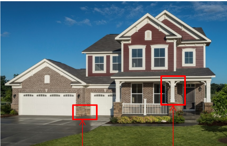
Masonry water table
